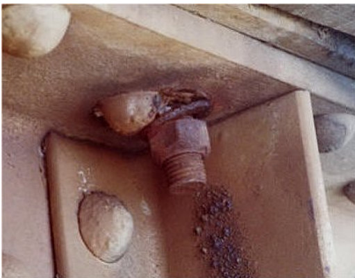
Traditional method of attaching ties to bridge deck. Repairs are needed weekly to retighten loosened bolts
