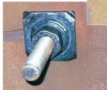
Using Locking fasteners on this bridge application, these bolts have been in use for over 3 years and have never needed re- tightening (Compared to every other week retightening or replacing hardware previously)
